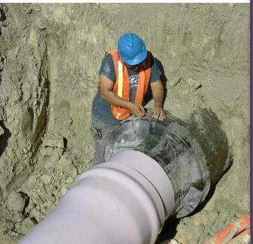
Top: Purple pipes are installed in a trench in the Bridgeland development. The pipes will carry non-potable water to irrigate common green spaces, saving millions of gallons of potable (drinking) water.
